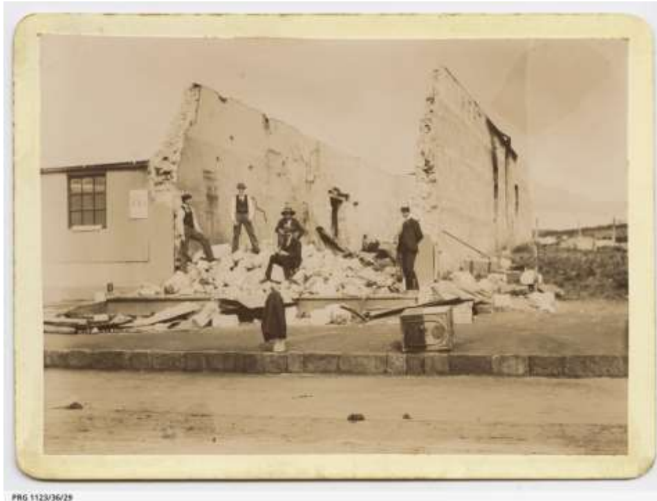
State Library of South Australia - Ruins of Macfarlane Brothers' store [PRG 1123/36/29], Men standing in the ruins of the Macfarlane Brothers general store, Port Lincoln, which was completely gutted by fire on 7 August 1900, causing £4,000 damage. 1900, Part of Bishop Family Collection.
