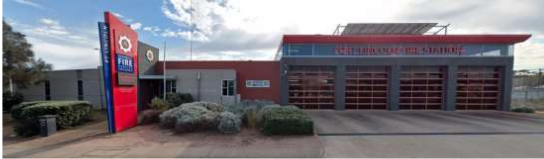
Port Lincoln MFS Fire Station 2023 Google Maps
