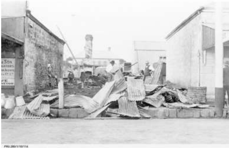
State Library of South Australia - Destruction caused by a fire on Tasman Terrace, Port Lincoln [PRG 280/1/10/114]. The aftermath of a fire which destroyed a building on Tasman Terrace, Port Lincoln, South Australia. 1914. Part of Searcy Collection
